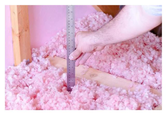
Fiberglass insulation is done mainly between joists, beams, and studs.
