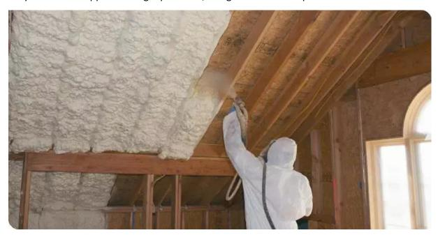
However, it should be kept in mind that this kind of insulation is much more expensive when compared to fiberglass insulation. In addition, it can also be a messy process. Also, the foam is made up of chemicals, which if inhaled can cause respiratory problems. Therefore, it is always advised to hire a handyman experienced in this task because you should make sure that the foam spread should be equal in every place.
