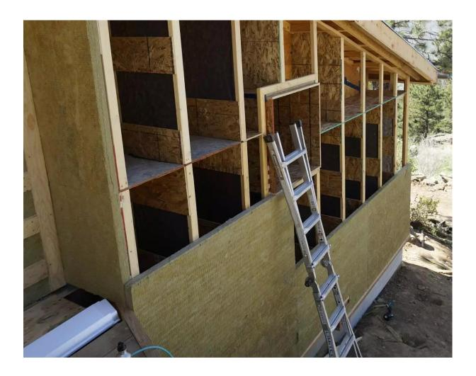
However, it is much more expensive when compared to fiberglass insulation and is also not found in the market commonly. One should also wear protective gear while installing it because the slivers in the loose fill are tiny enough to get into your nose and can also cause cancer in the lungs.
